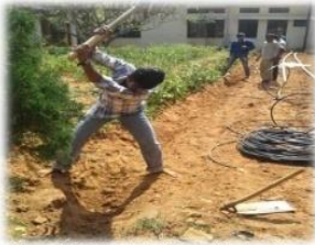
Trench for installation of irrigation pipes
