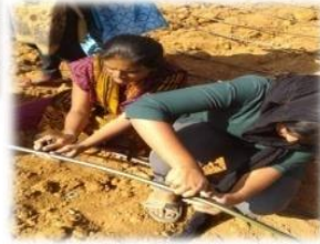
Fixing of Drippers to lateral pipes
