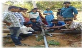
Connecting Disc filter to submains
